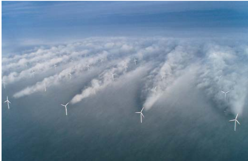
Figure 5: Downstream wake and turbulence effects
